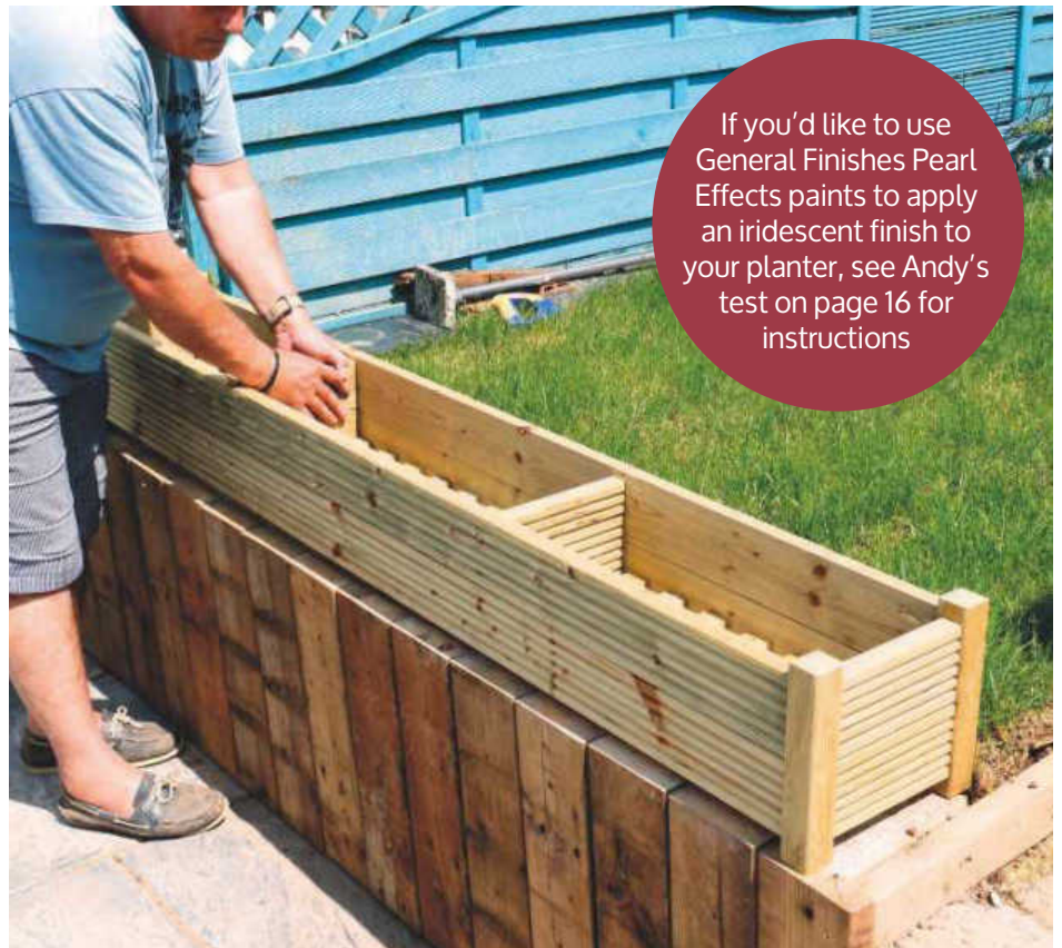
STEP 15. A couple of dividers help keep the sides from bulging out
